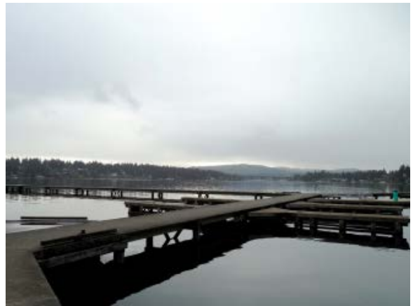
Photo 6A – Large pier
