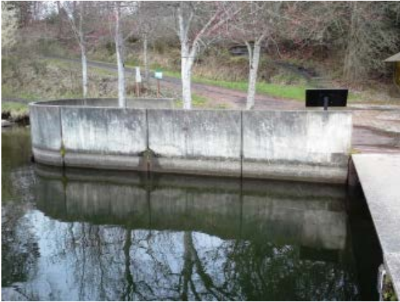
Photo 1A – Concrete bulkhead
