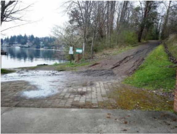
Photo 3A – Gravel maintenance road
