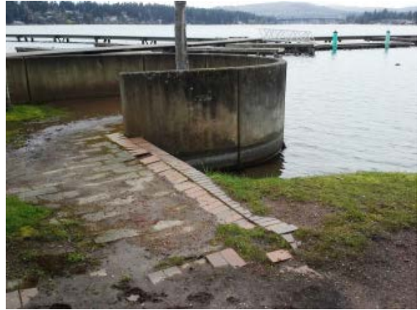
Photo 2A – Brickwork adjacent to bulkhead
