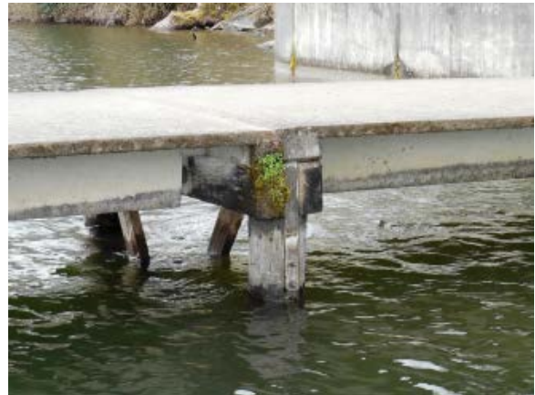
Photo 8A – Typical pier construction
