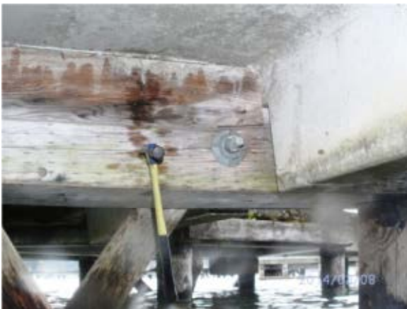
Photo 17A – Precast "T" and timber cap beam
