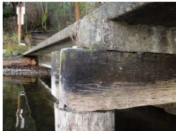
Photo 24A – Pile cap to pile connection (small pier)
