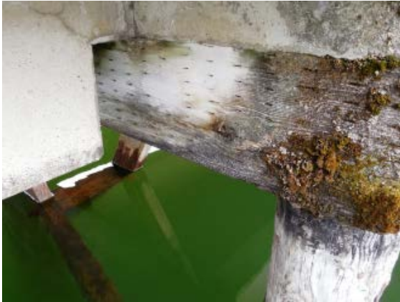
Photo 13A – Treated cap beam at pile
