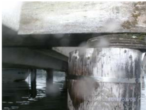
Photo 18A – Plywood shims between cap and pile
