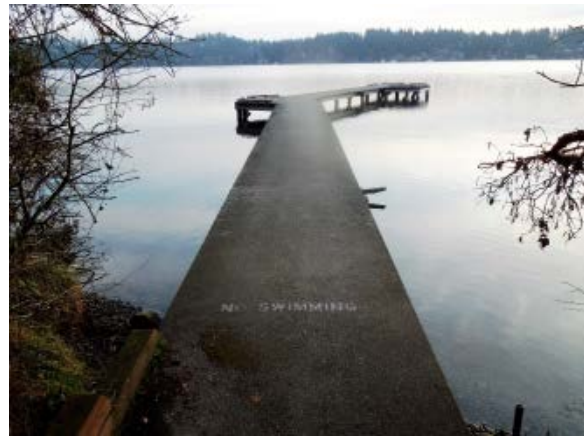
Photo 22A – Small pier
