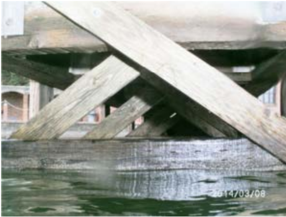
Photo 19A – Diagonal bracing
