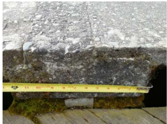
Photo 10A – Pier slab over support
