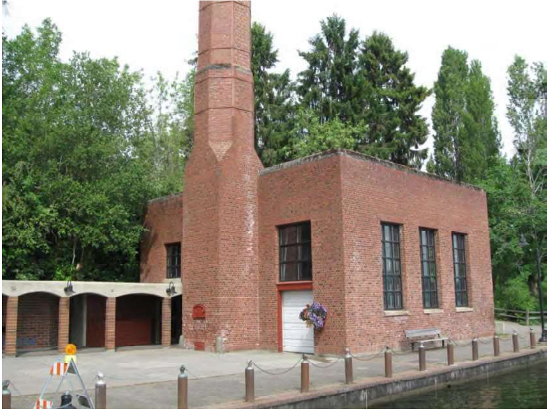
Figure 3: View from dock showing 1974 restroom addition
