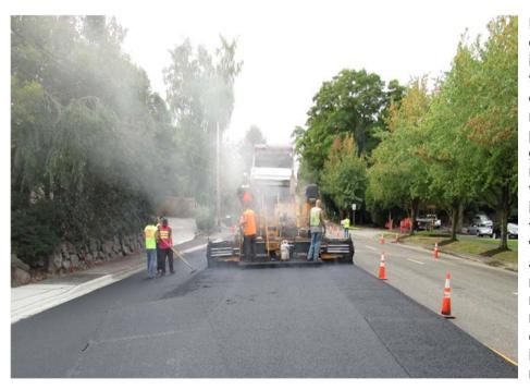
Major elements of this capital project included: repairs to the roadway's storm drainage system, repair of failed pavement areas, grinding of the entire roadway to remove the paving lift placed in 1991, resurfacing of the entire roadway with a 3" hot mix asphalt overlay, and new pavement markings. The roadway's width, lane configuration, and intersection layouts remained unchanged.
