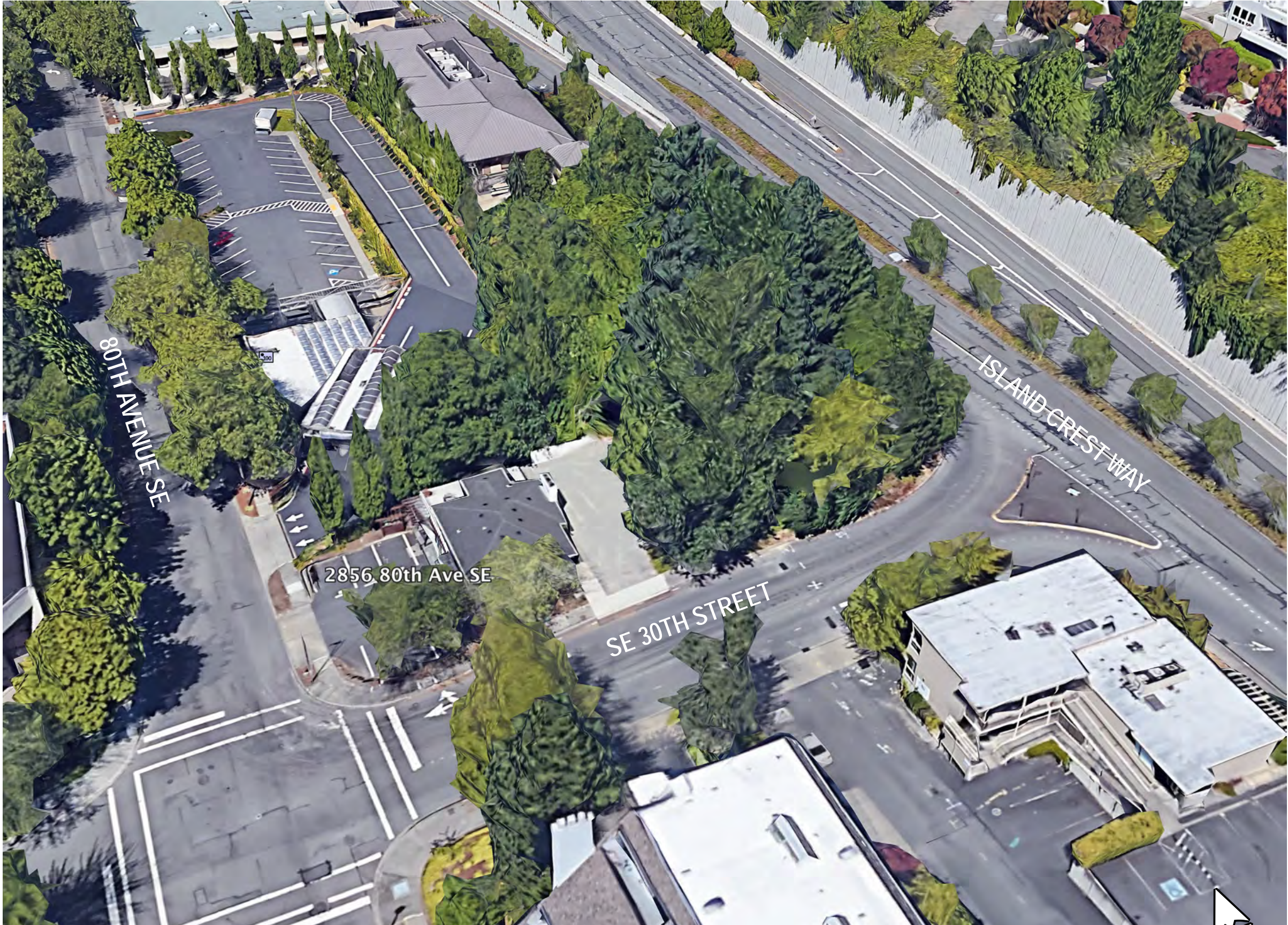
AERIAL VIEW OF SITE LOOKING NORTHEAST
