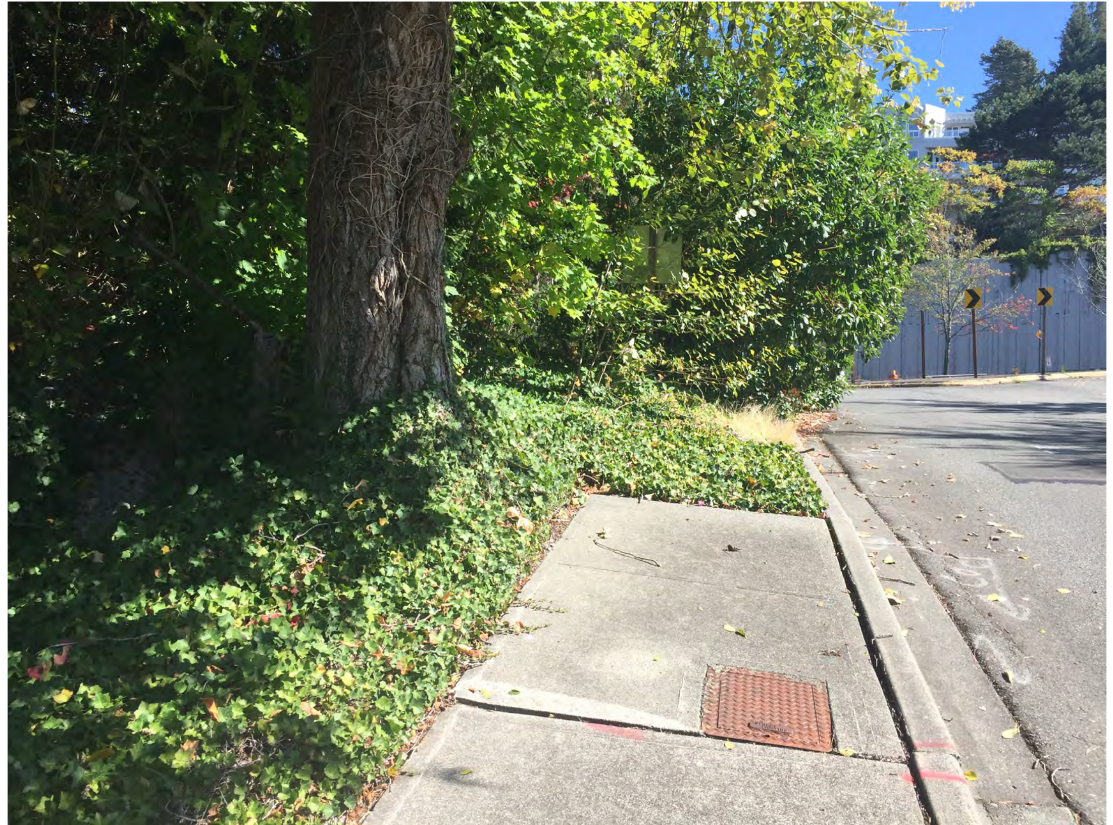
VIEW OF EXISTING SIDEWALK ON THE EAST END OF SE 30TH STREET AS IT MEETS ISLAND CREST WAY
