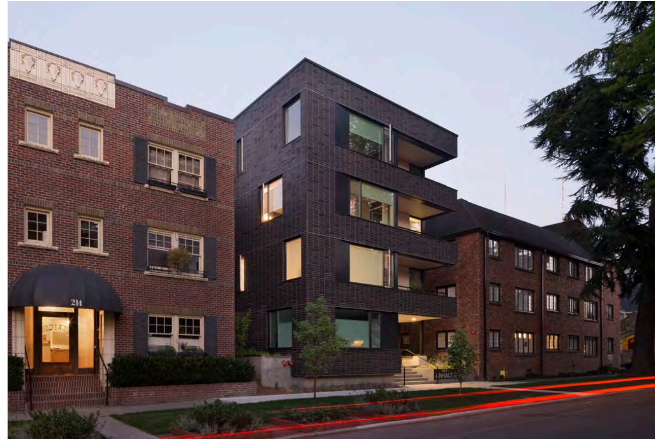
Anhalt Apartment Renovation and Addition [with East Seattle Partners] Seattle, WA
