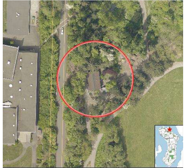
90.05.0009 LUTHER BURBANK CARETAKER FACILITY REPAIRS
