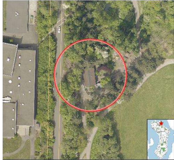
90.05.0009 LUTHER BURBANK CARETAKER FACILITY REPAIRS
