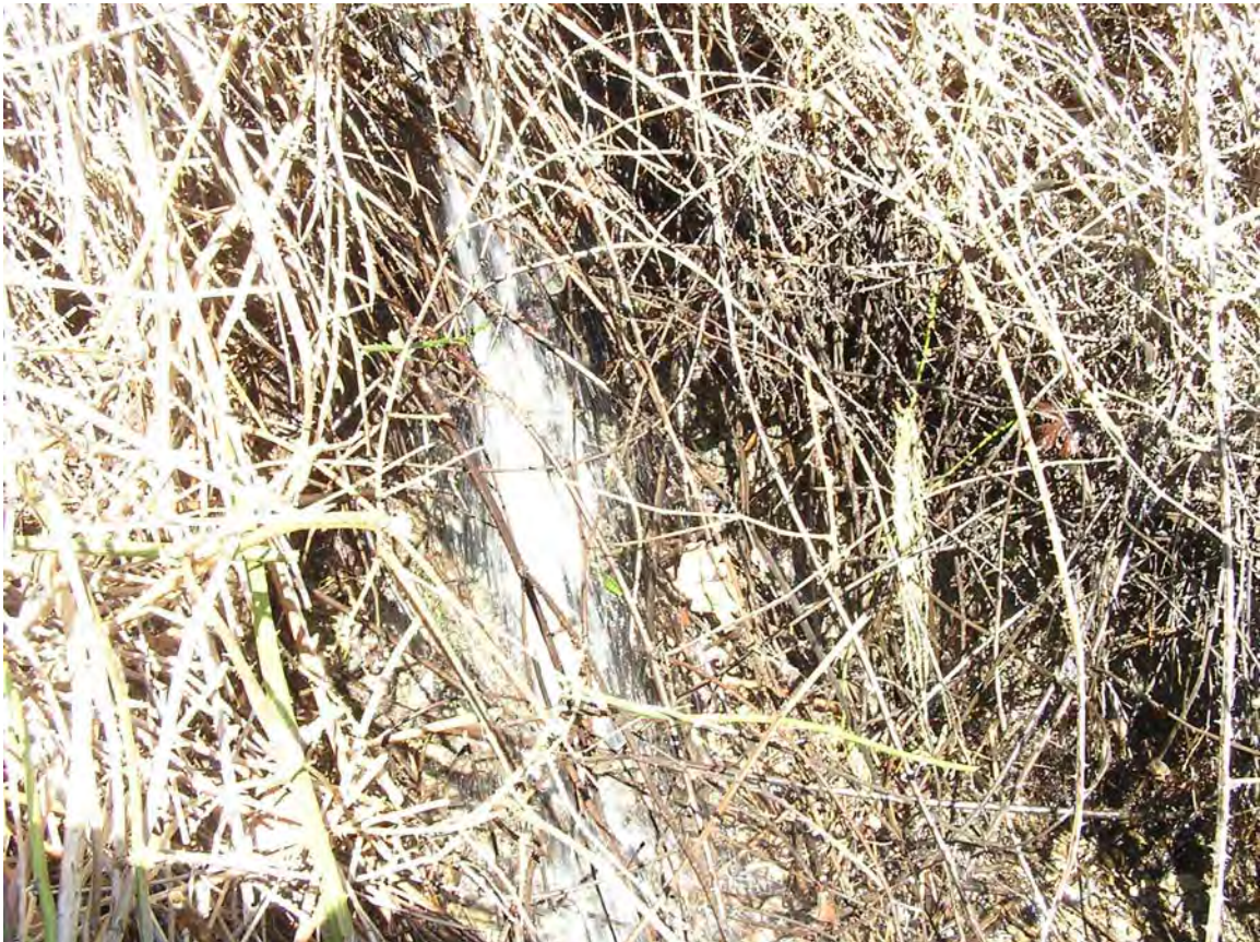
Flow from Pipe Outlet 3/3/2006
