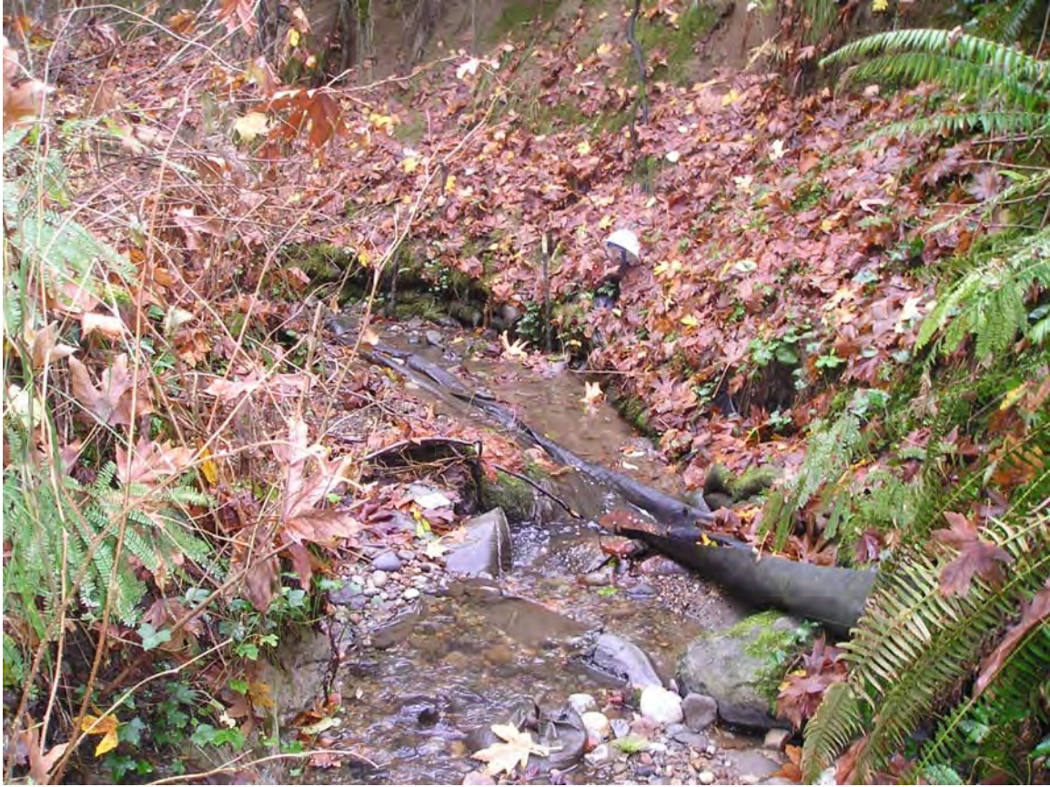
Looking Downstream at Sandbagged Bank 1/5/2006
