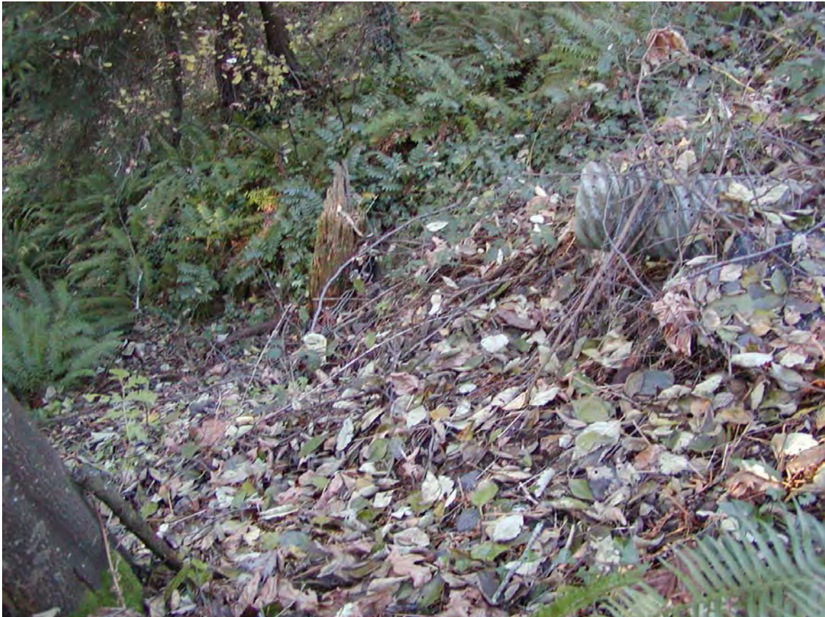
Culvert Outfall on Steep Slope 12/8/2005
