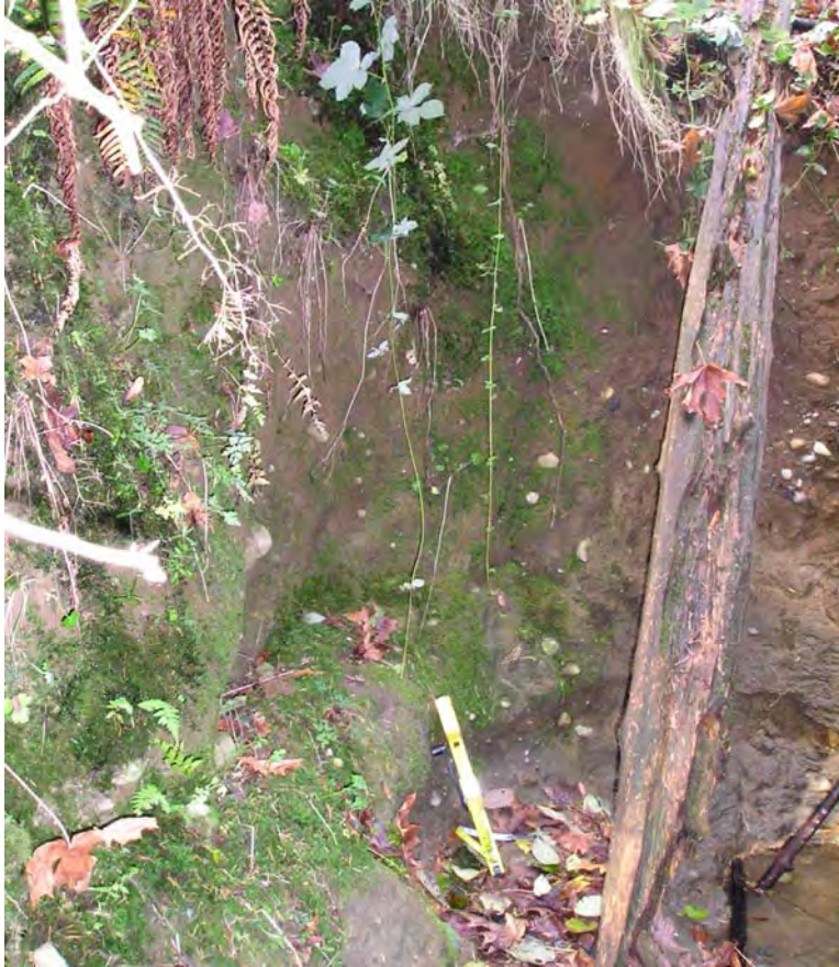
Looking Upstream at Headcut 1/5/2006
