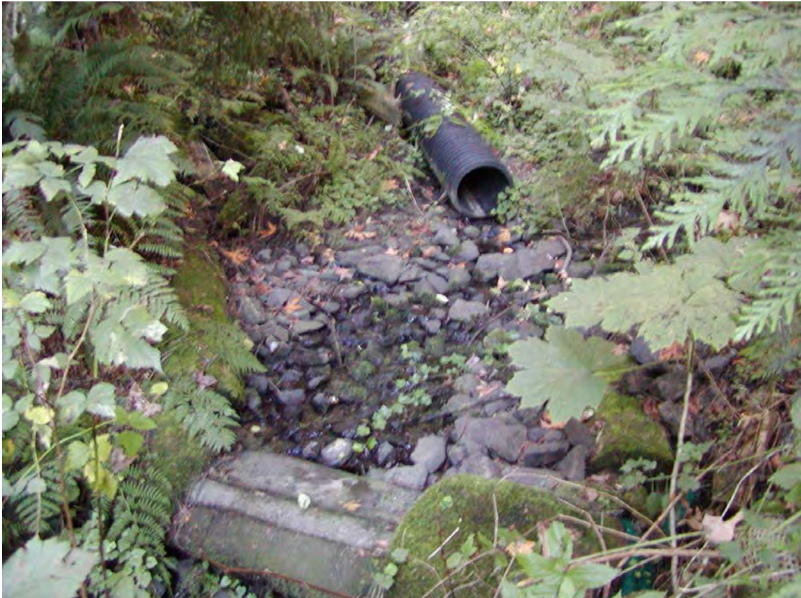
Looking Upstream at 18" Corrugated PE Pipe Outlet 9/28/2005
