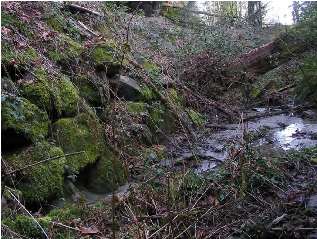
Looking Upstream. Rock Protection on left. 3/3/2006
