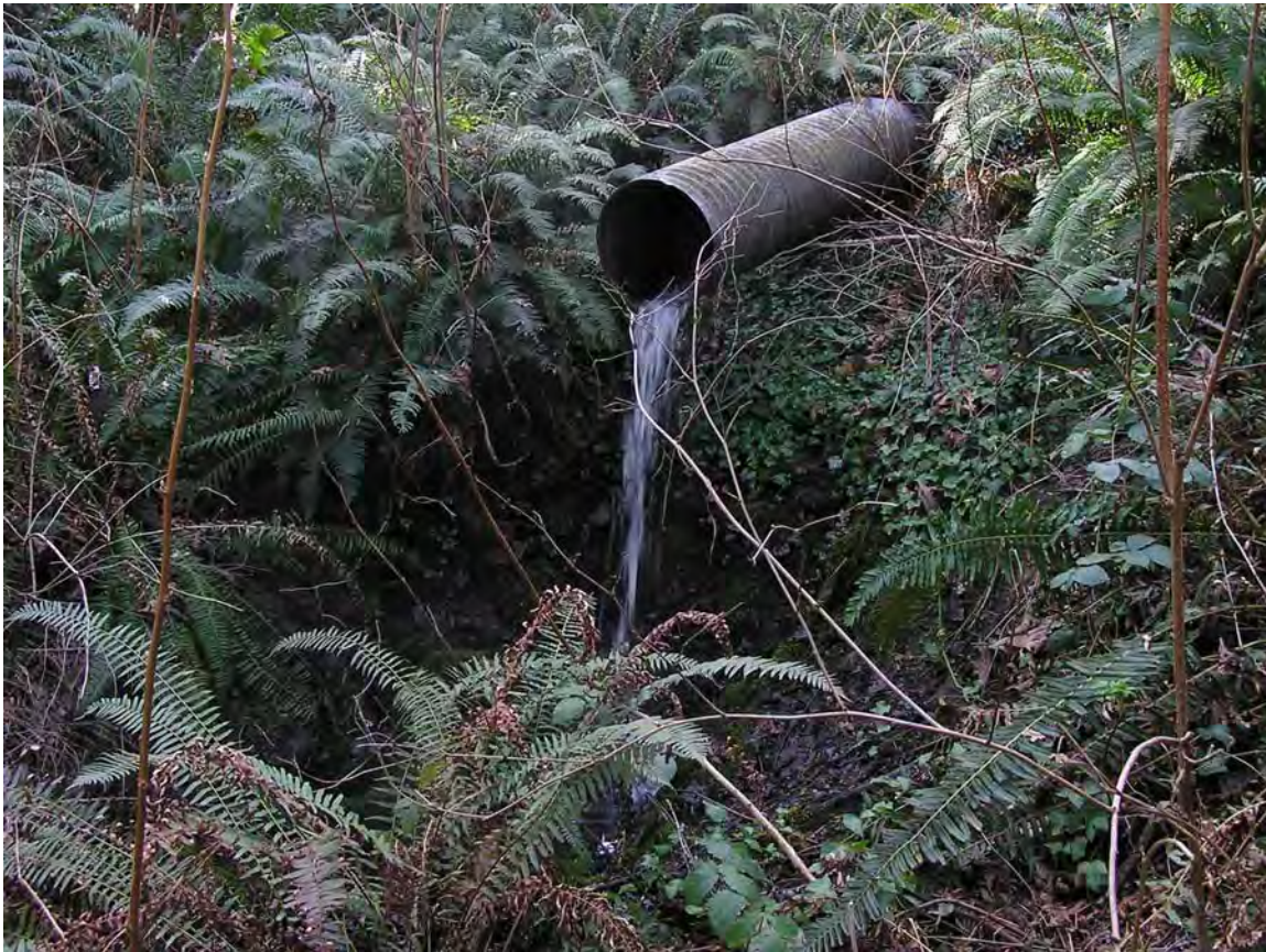
Looking Upstream at Culvert Outlet 3/3/2006
