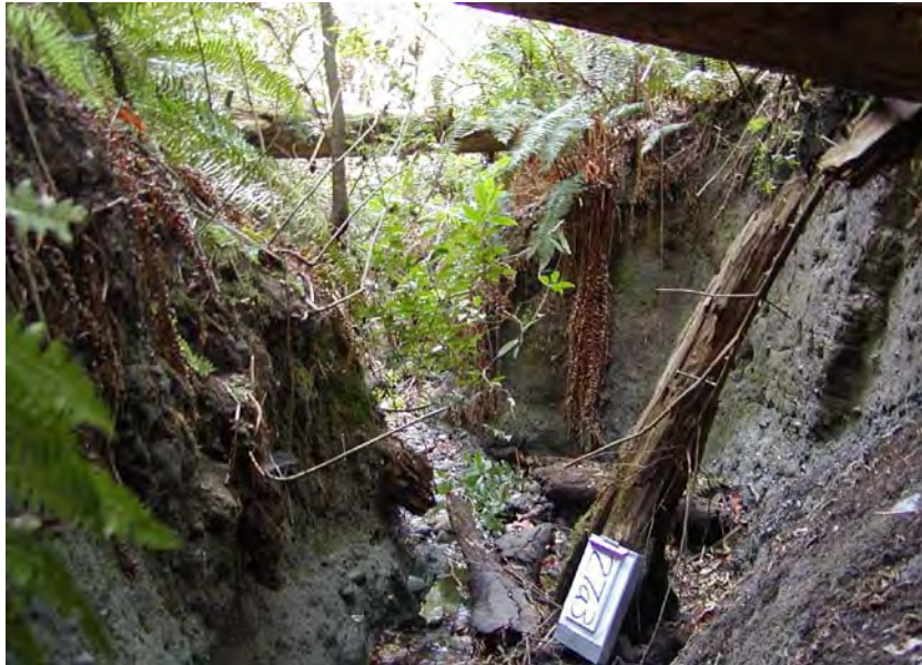
Project 27a.3: Looking Downstream - 9/28/2006
