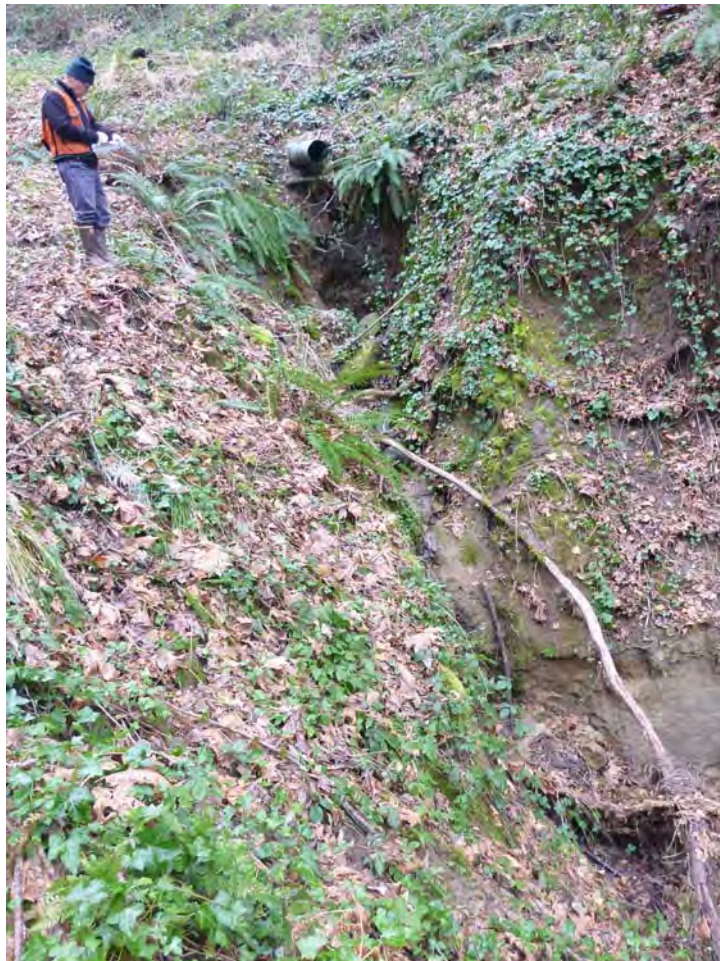
Looking Upstream at Total 25' Vertical Drop 03/09/2012
