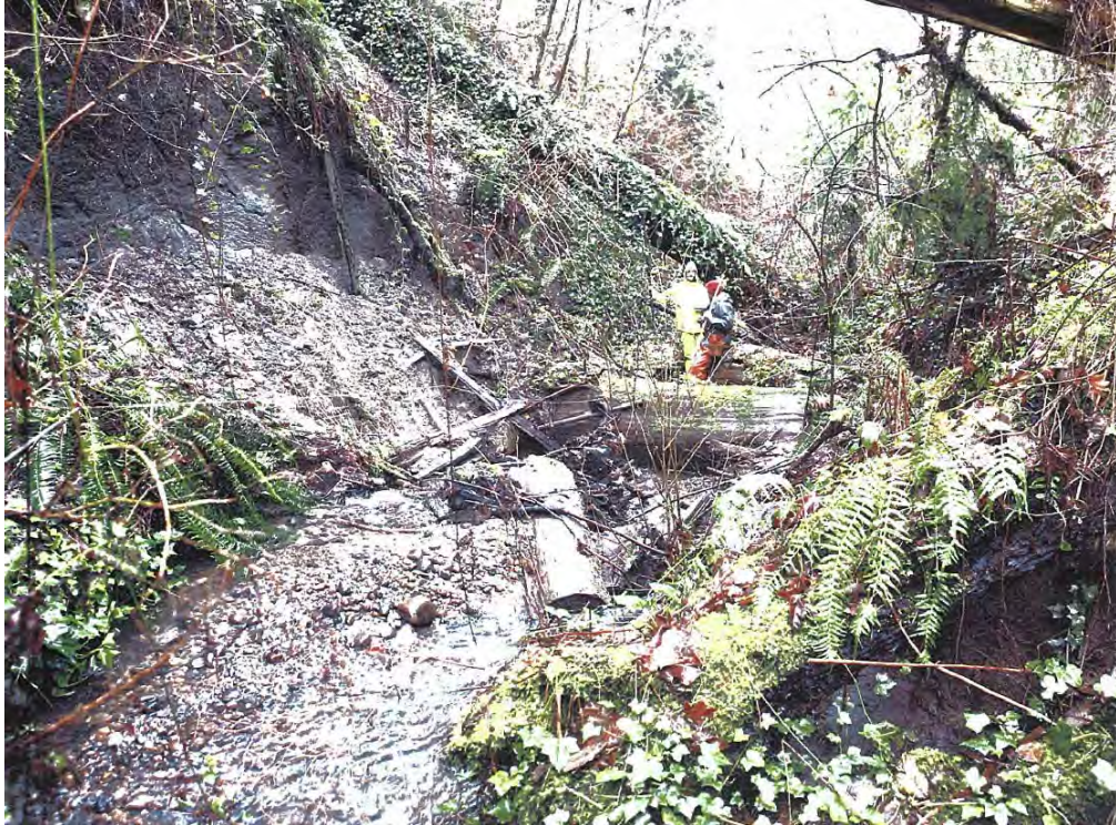
Project 6.5: Failed Log Weir Station 33+20 2/15/2011
