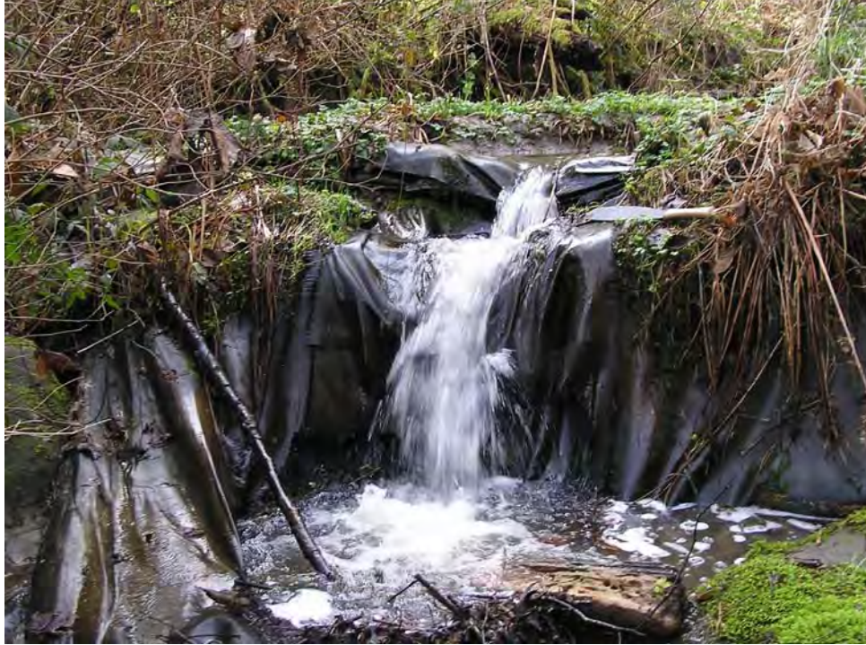
Looking Upstream at 3' High Sandbag and Geotextile Dam 9/28/2005
