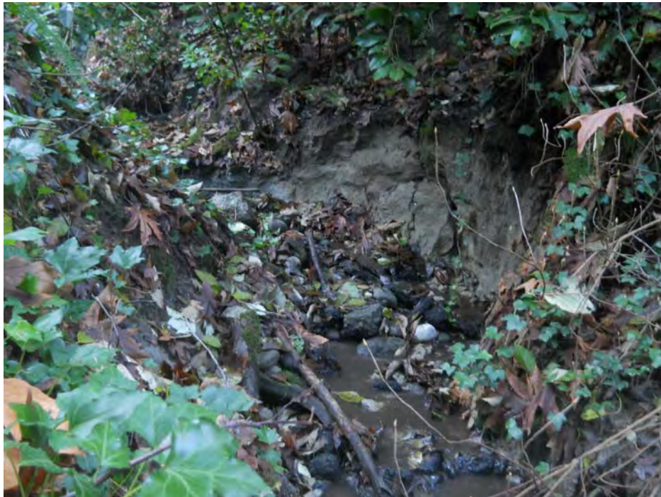
Looking Upstream at Recent Bank Erosion 12/22/2011
