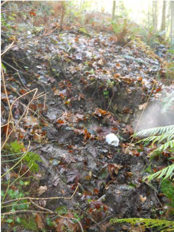
Recent Slope Toe Failure from Bank Erosion 12/22/2011
