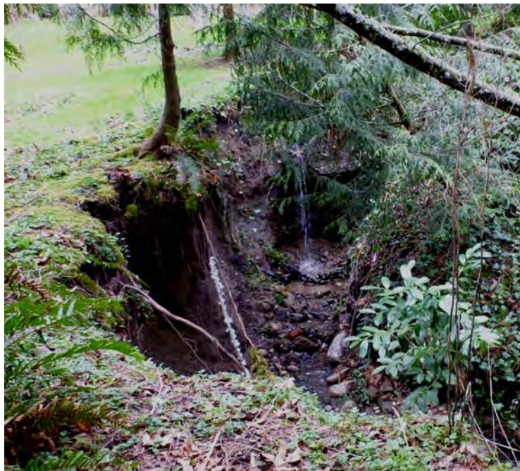
Project 27a.11: Looking Upstream 03/09/2012
