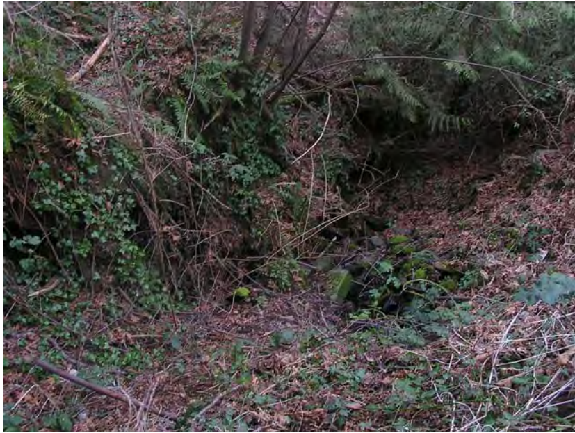
Project 4.2: Looking Downstream at Outlet 9/24/2005
