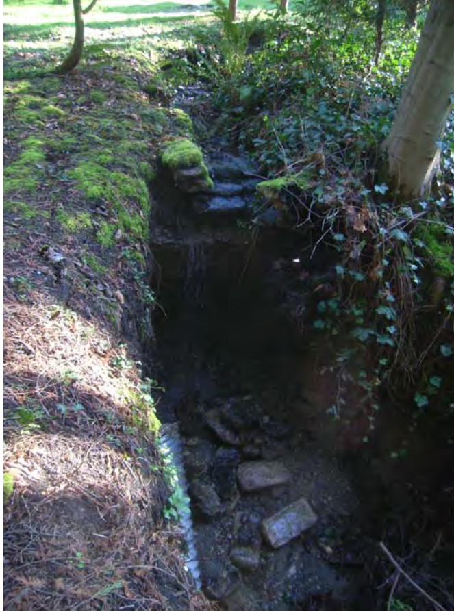
Project 27a.11: Looking Upstream 03/17/2010
