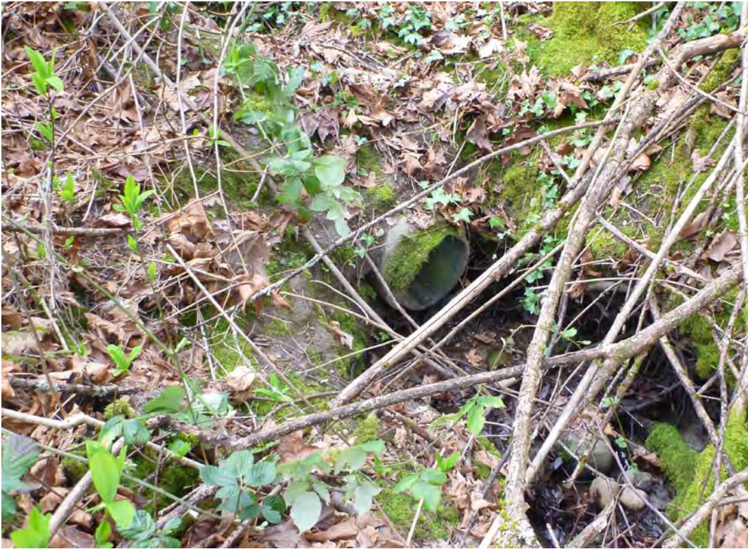
Outfall of 12" reinforced concrete pipe under West Mercer Way 03/09/2012
